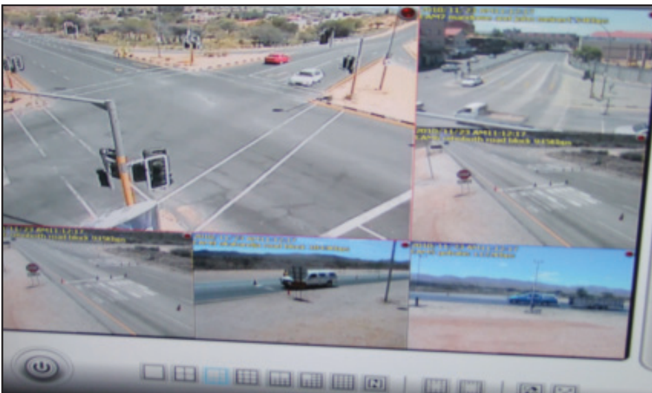
The City Police are now able to monitor movements and detect criminal activities easily, thanks to the installations of CCTV at various places in Windhoek.
