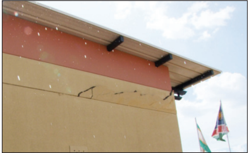
This crack is too wide to be fixed as it runs through the wall.
